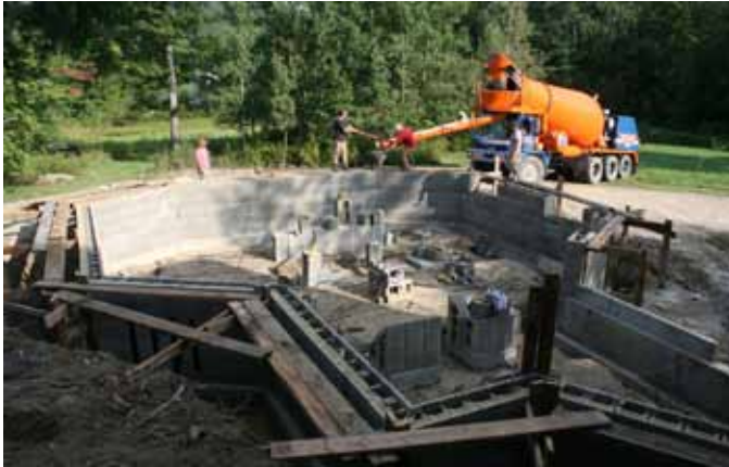
Building the walls of the lower level; the walls are made of 14-inch thick insulated blocks that consist of concrete-bonded recycled waste wood fibers. Once the blocks are stacked, the core is filled with concrete.
