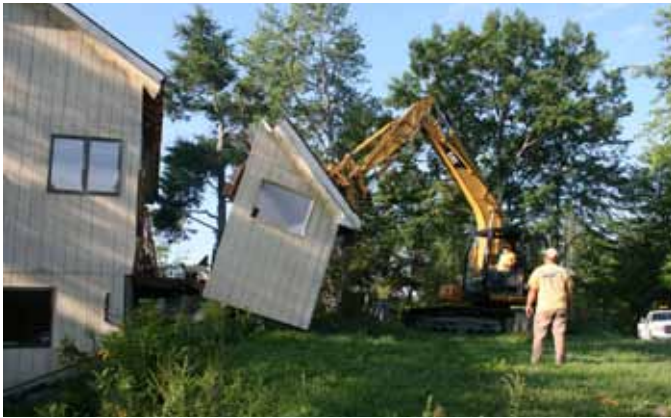
Removing the previous entryway to our building on August 13
